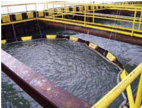
First Sheen Boom deployed in the out-fall of a major power plant.
