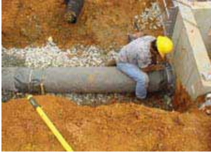
Water gate install.
