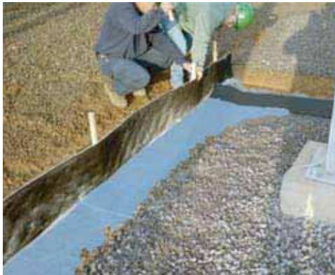
Boom with flap supported by stake
